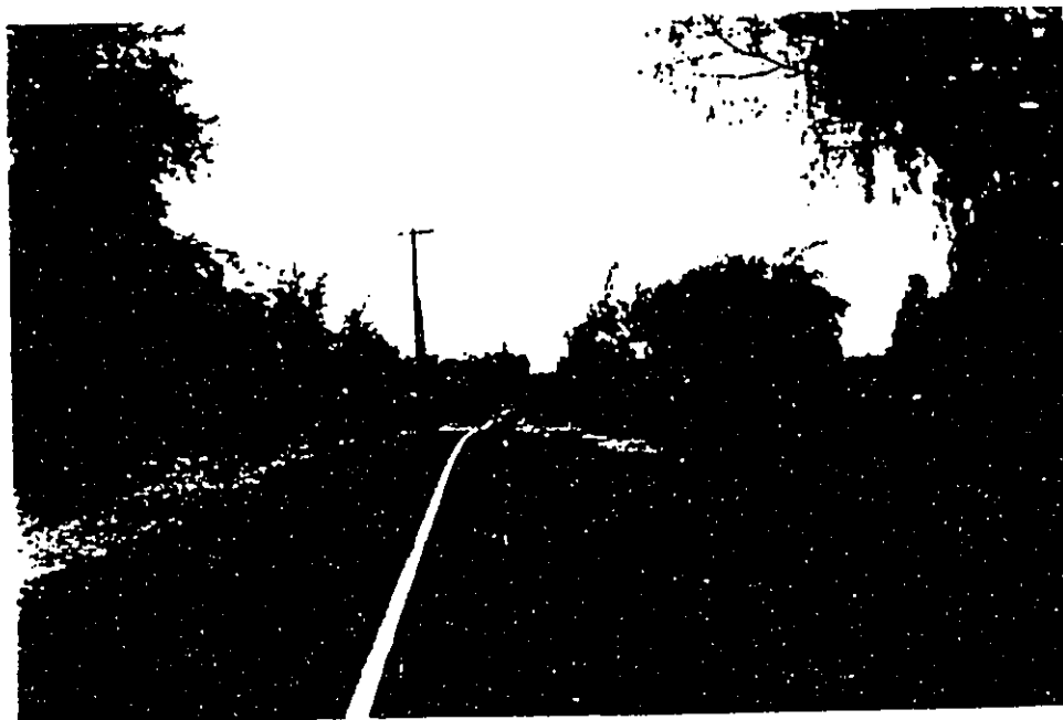
Figure 14 Pole Placements Within Highway #137 Right-of-Way
