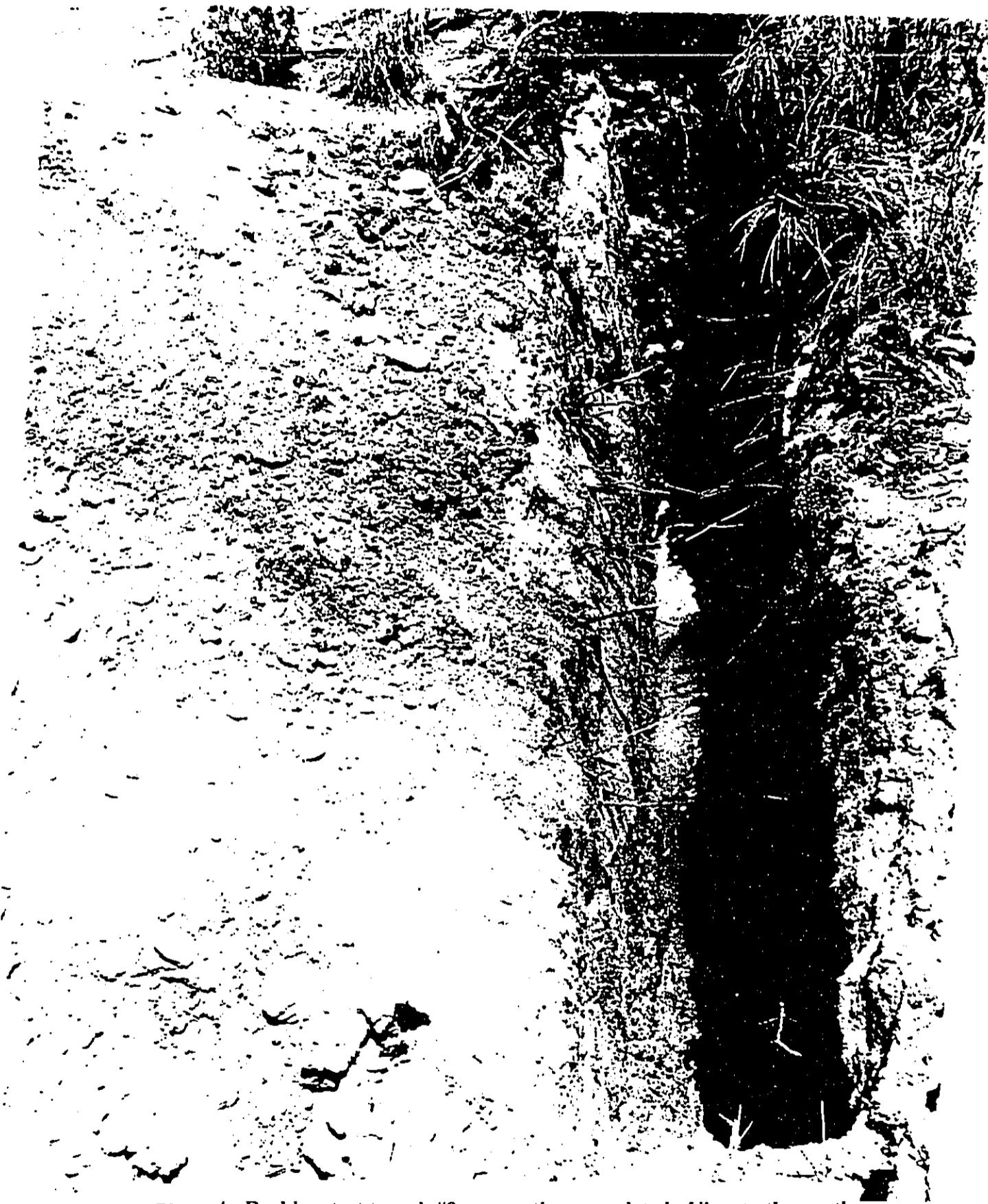
Photo 4 - Backhoe test trench #9, excavation completed. View to the north.
