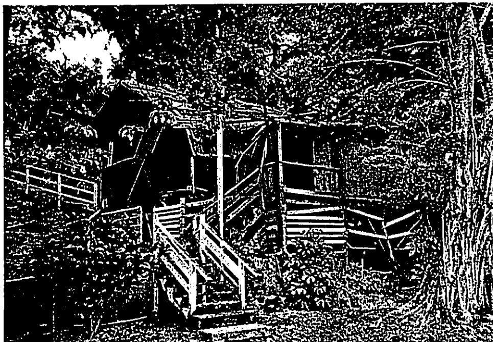
Photo 1. Collapsing wooden structure, ca. the late 1930s.
