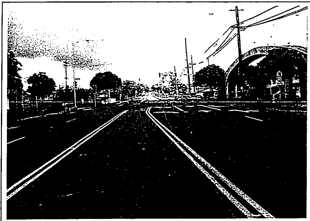
Waimano Home Road at Moanalua Road (facing north)
