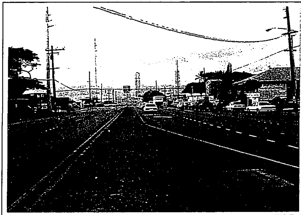
Kamehameha Highway approach to Waimano Home Road (facing west)
