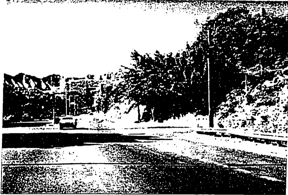
Figure ES-1. Kalaniana'ole Highway at Kapaa Quarry Road Looking West
