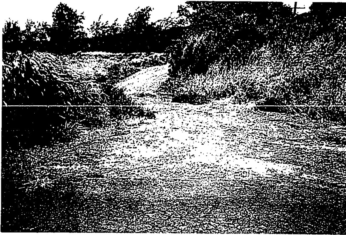
5. View south of proposed pipeline route start, booster location.
