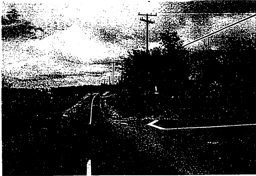
Photo 3-4 Pole Placements Within Highway #137 Right-of-Way
