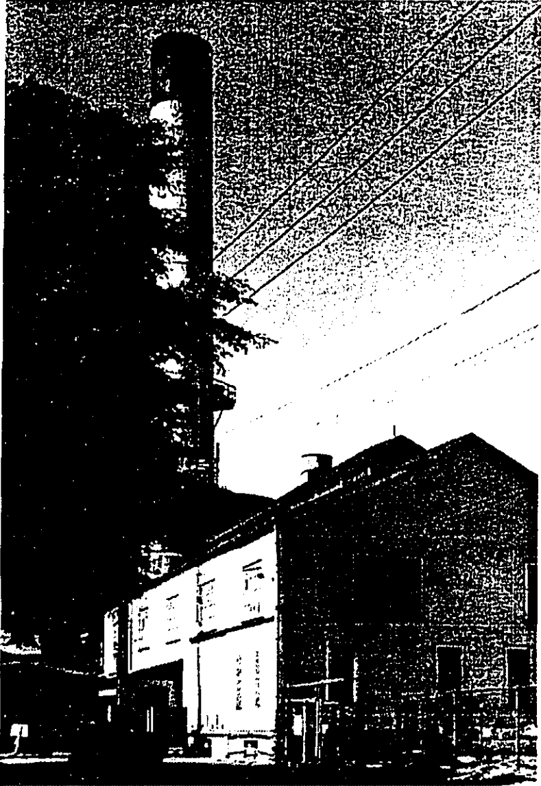
① Mill Smokestack and Generator Building
