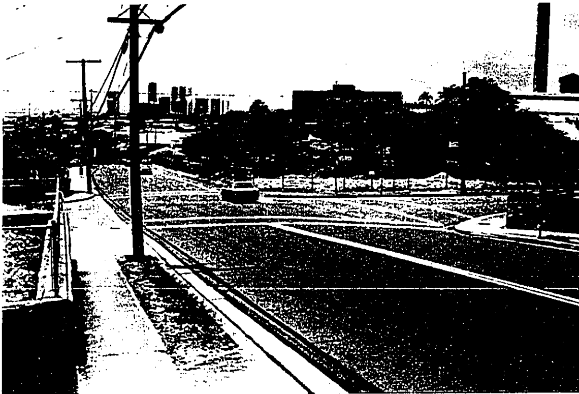
Figure ES-4. Ulune Street with Kulawea Street (looking northwest)
