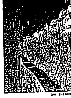
After the Little Patuxent River streambank is excavated, fiber branches from willow and dogwood trees are installed so that their legs extend over the stream. The branches are anchored in place with stakes and covered with soil. (The temporary diversion wall was installed to prevent erosion during construction.)
