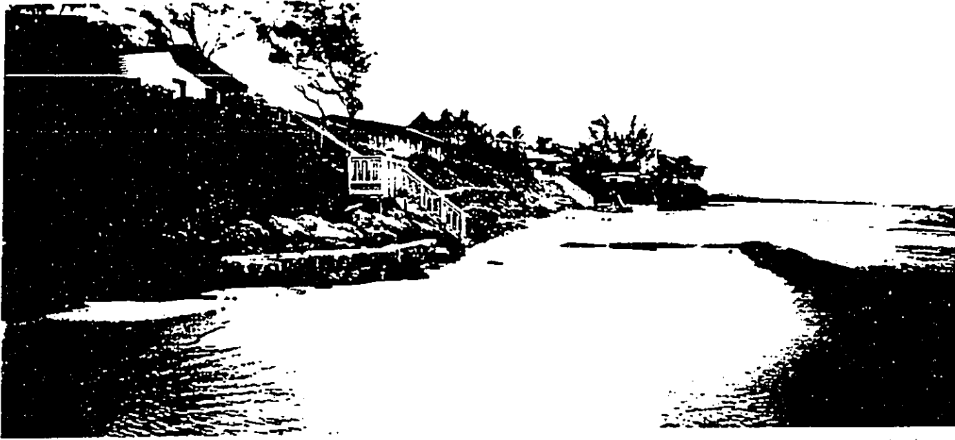
Photo No 3. This view of the revetment at TMK 5-5-02:86 shows the relationship of the collapsing wall at the foot of the revetment and boulders behind it.
