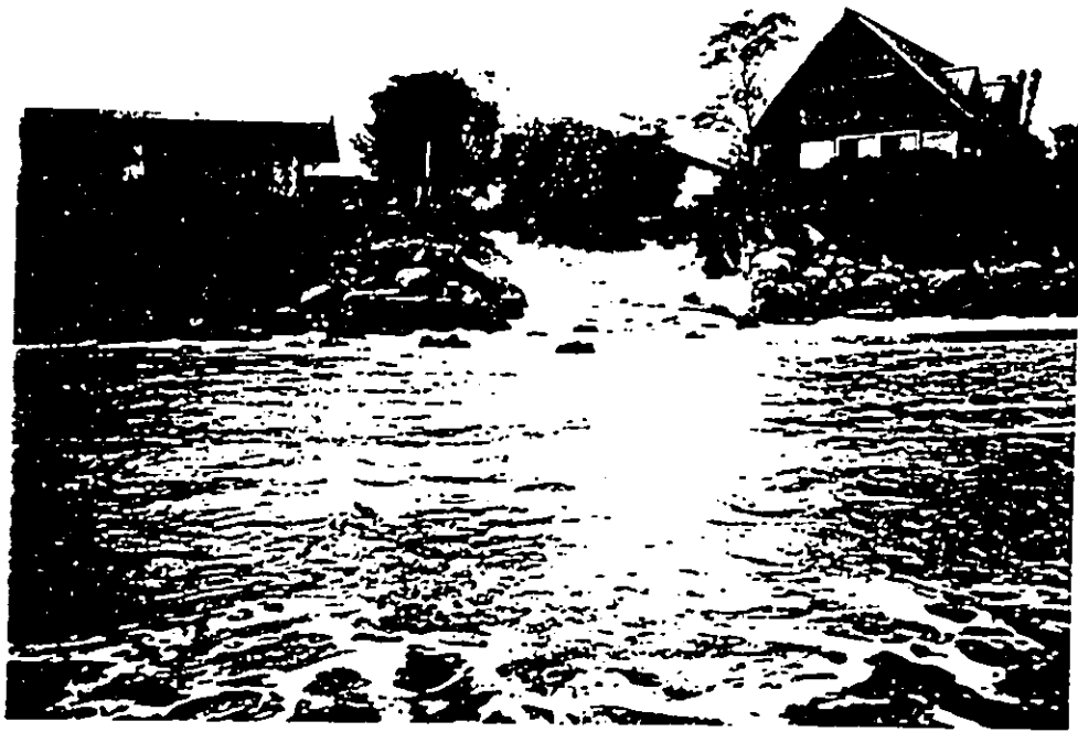
Photo Nos. 14 & 15. This gap in the shoreline revetments is for the 10-foot wide shoreline access for TMK 5-5-02:67. TMK 5-5-02:34 is on the left and TMK 5-5-02:32 is on the right. This is the only break in shoreline protection to the north of the subject property.
