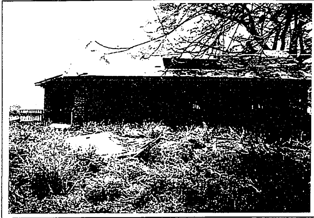
FIGURE 10: NORTH SIDE OF BUILDING NO. 3987. VIEW TO SOUTH.
