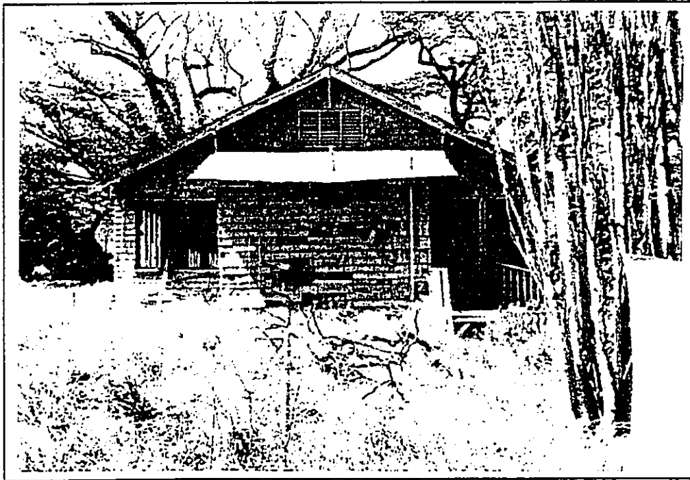
FIGURE 11: EAST SIDE OF BUILDING NO. 3987. VIEW TO WEST.
