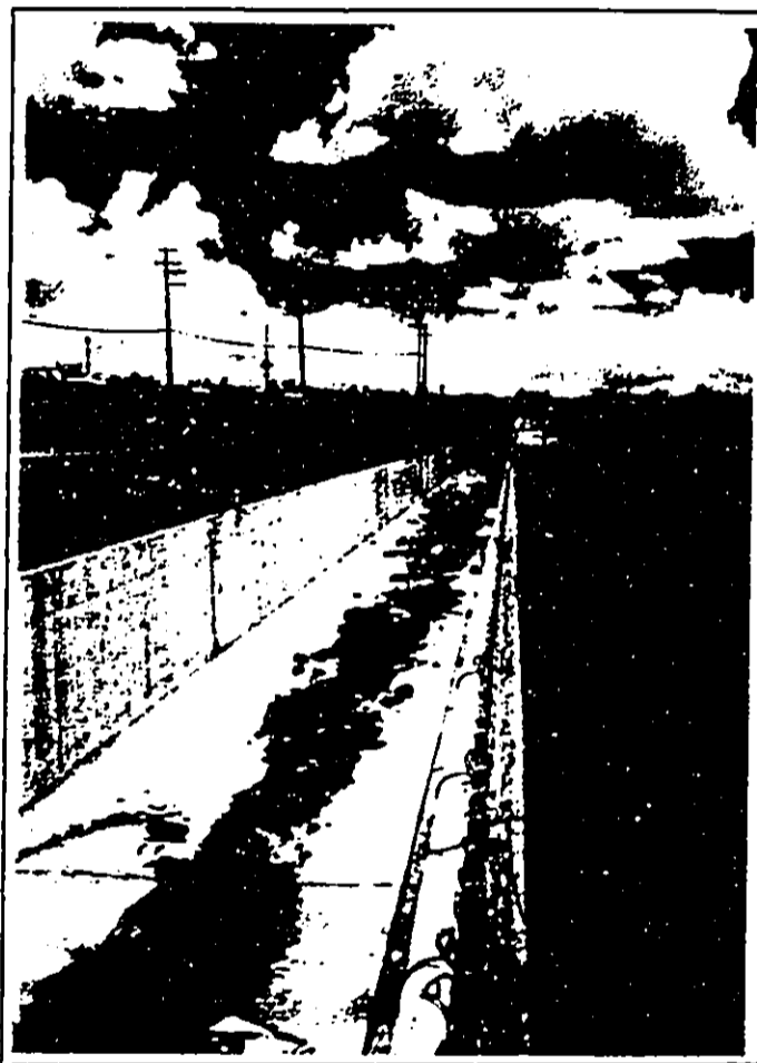
Photo G: Drainage channel bordering the property to the north; looking east.
