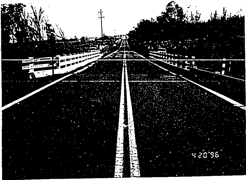
Popoo Bridge, Looking North Along Hawaii Belt Road
