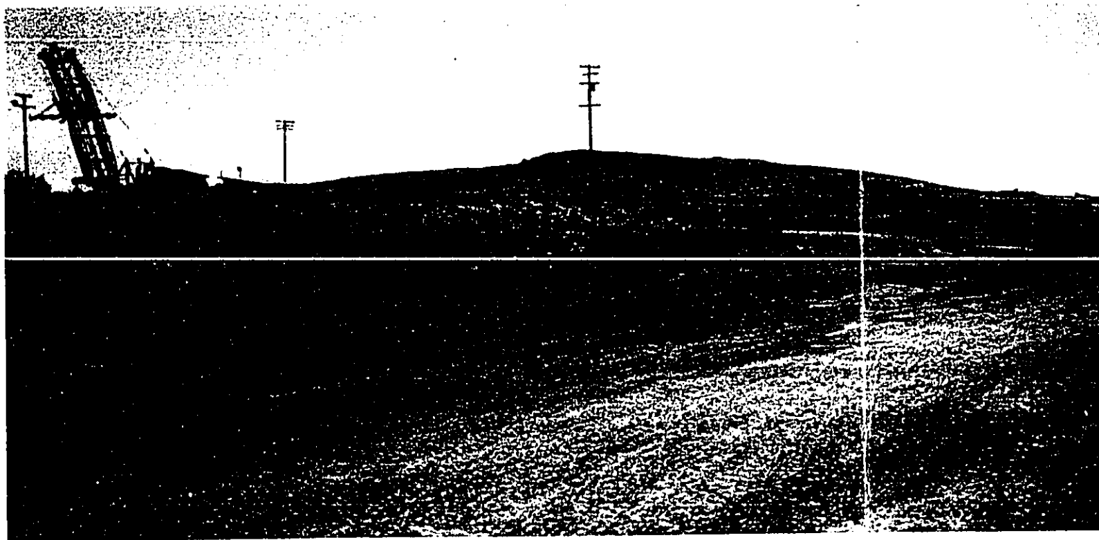
2) VIEW LOOKING SOUTHEAST TOWARDS EXISTING 1.5 MG TANK SITE
