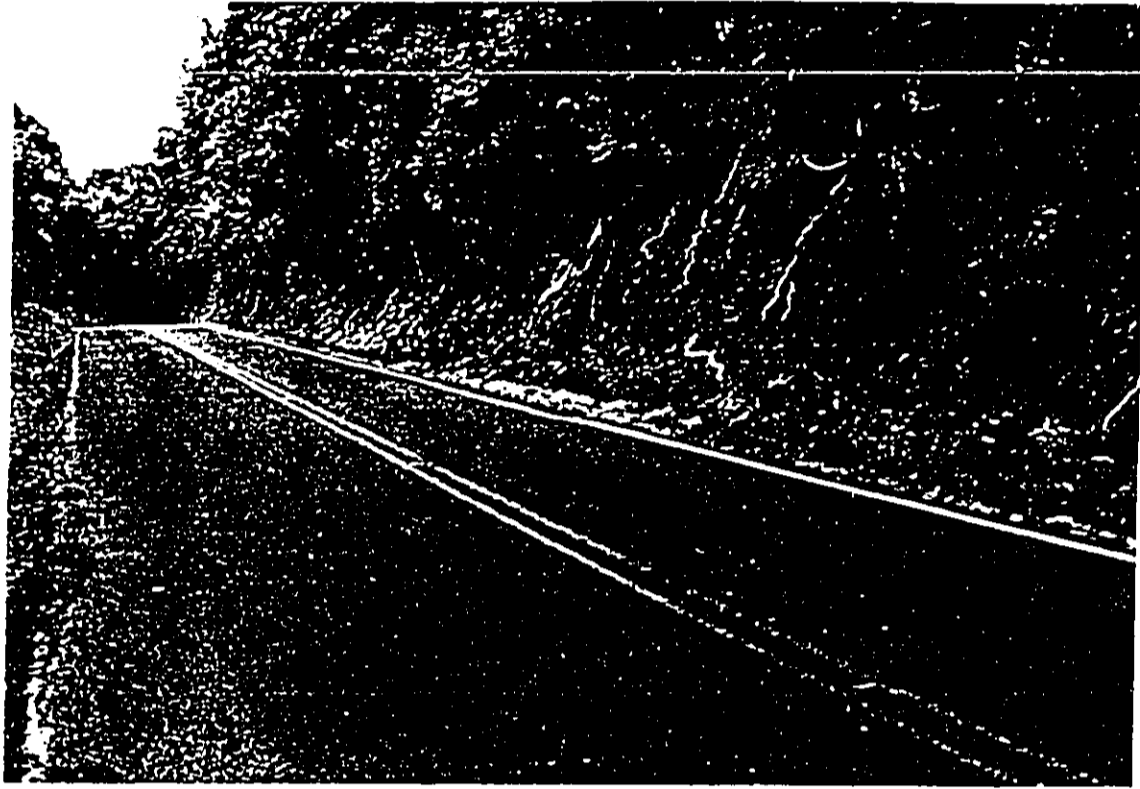
Figure 10 Central portion of Auloa Road right-of-way study area showing cut in ridge to create road alignment; view northeast
