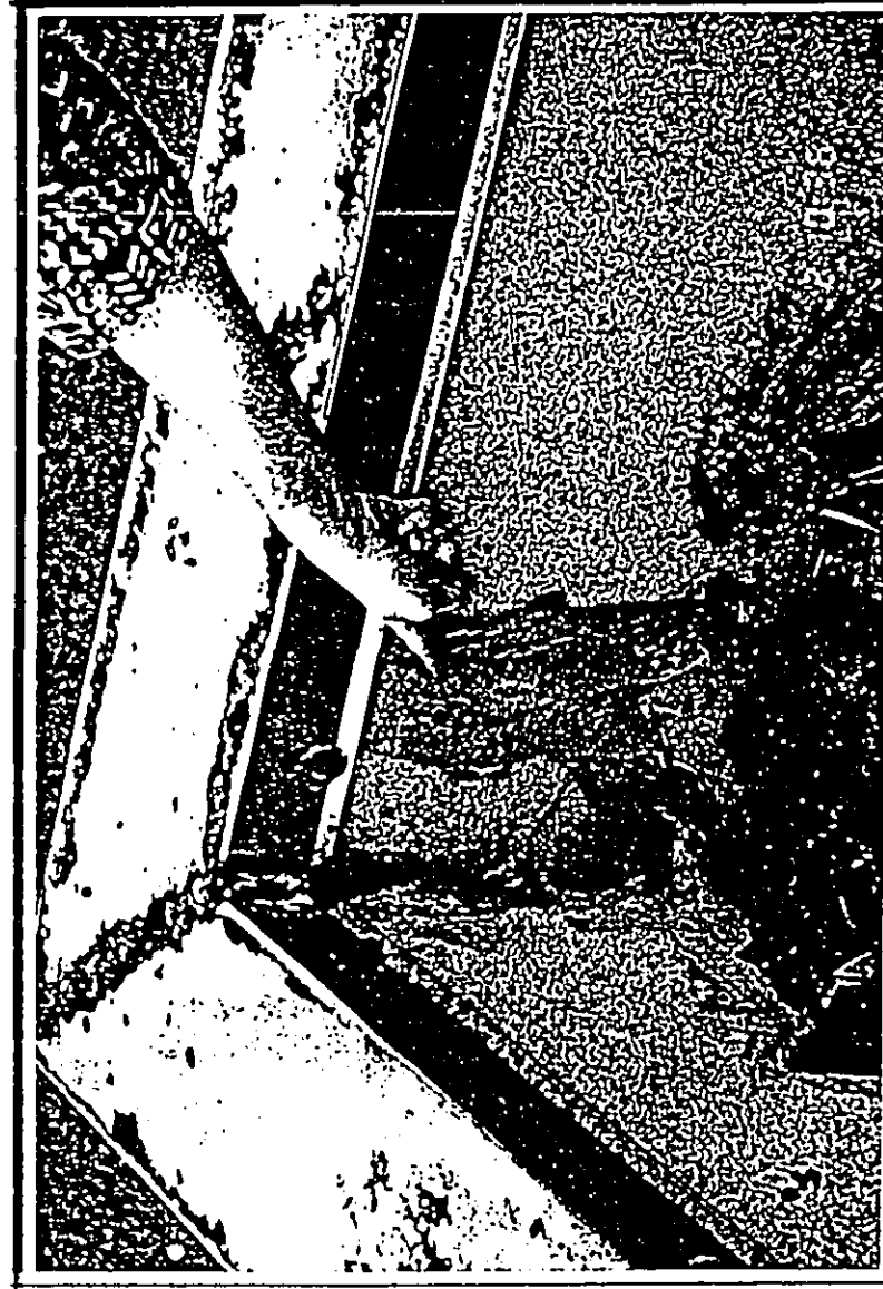
Gray caulk on vertical shingles of Turbine Building roof perimeter.
