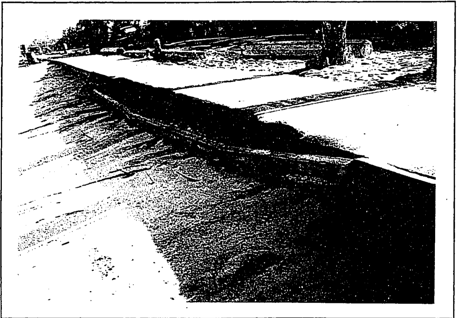
Figure 1.3: Photograph taken 1/11/96 after a large storm wave event showing undermining of the bike path on the berm crest.
