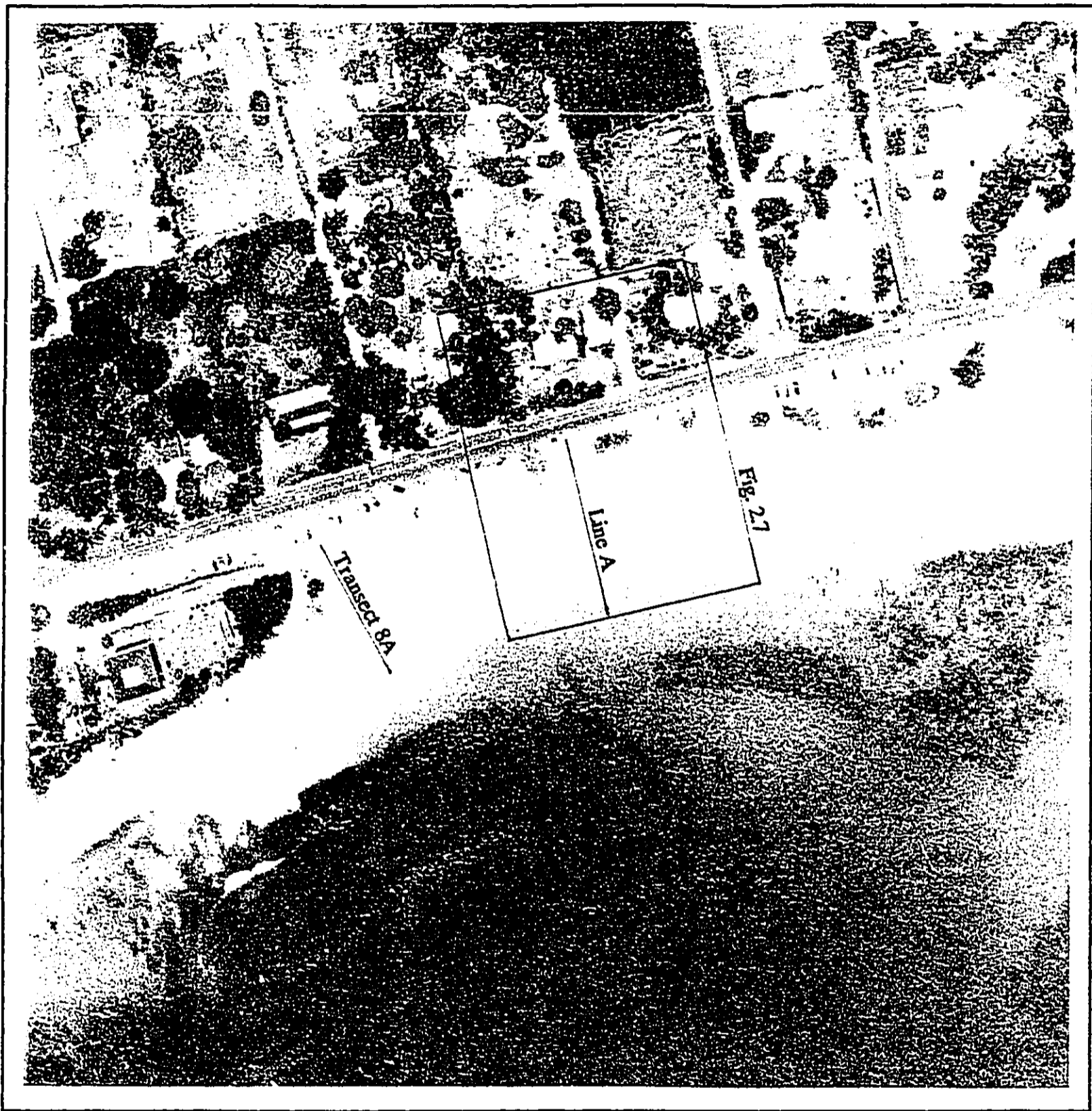
Figure 1.2: Aerial photograph of the project site (September 11, 1995, R.M. Towill Corp.)
