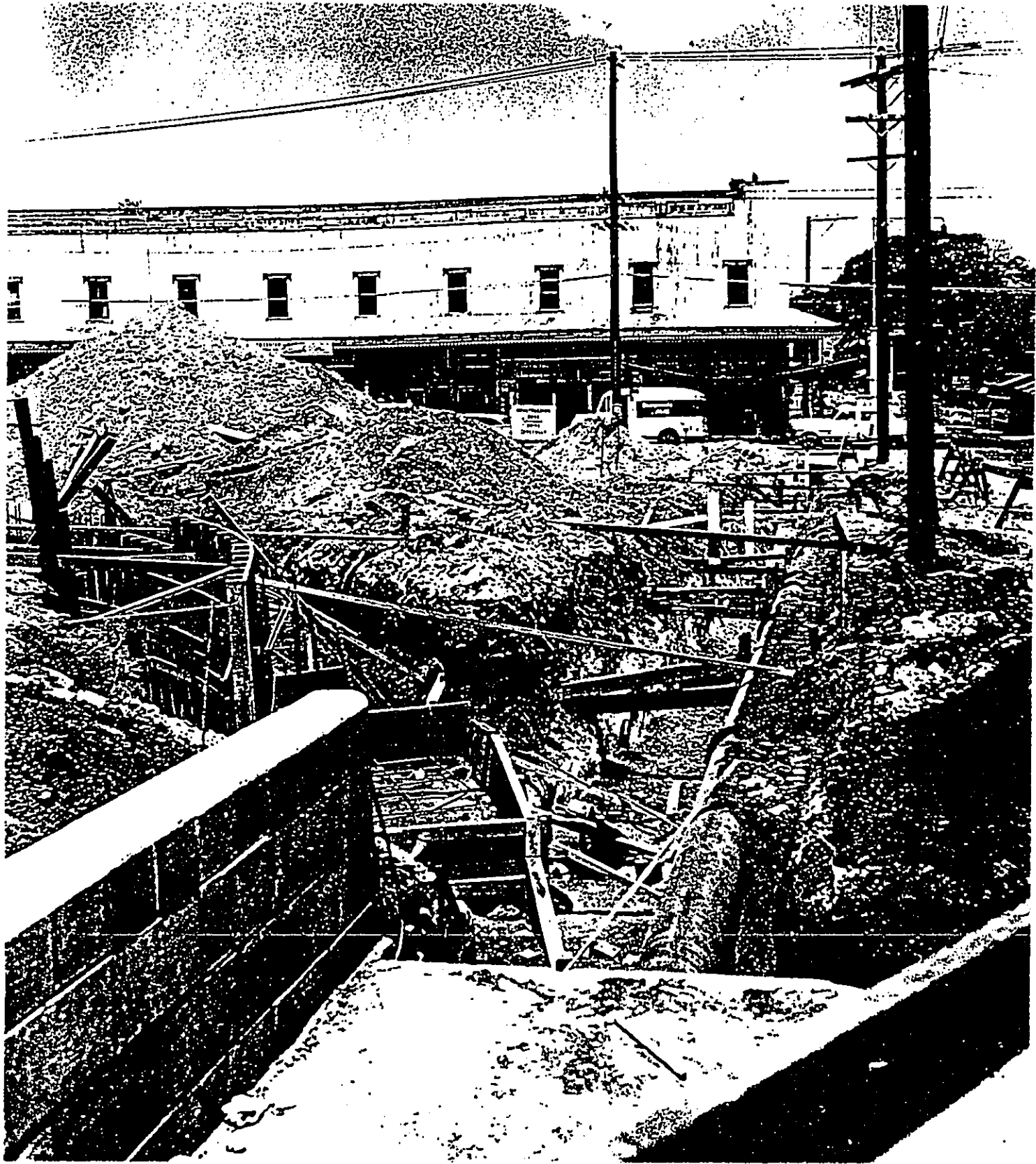
Figure 15 Photograph (August 30, 1959) showing excavation at corner of Kukui St. (on right) and Fort St. (in background) within present project site (Bishop Museum Archives)
