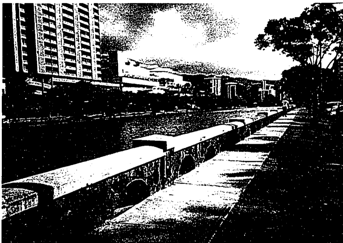
Figure 7: (bottom) Ala Wai Canal, stairs, looking SW.
