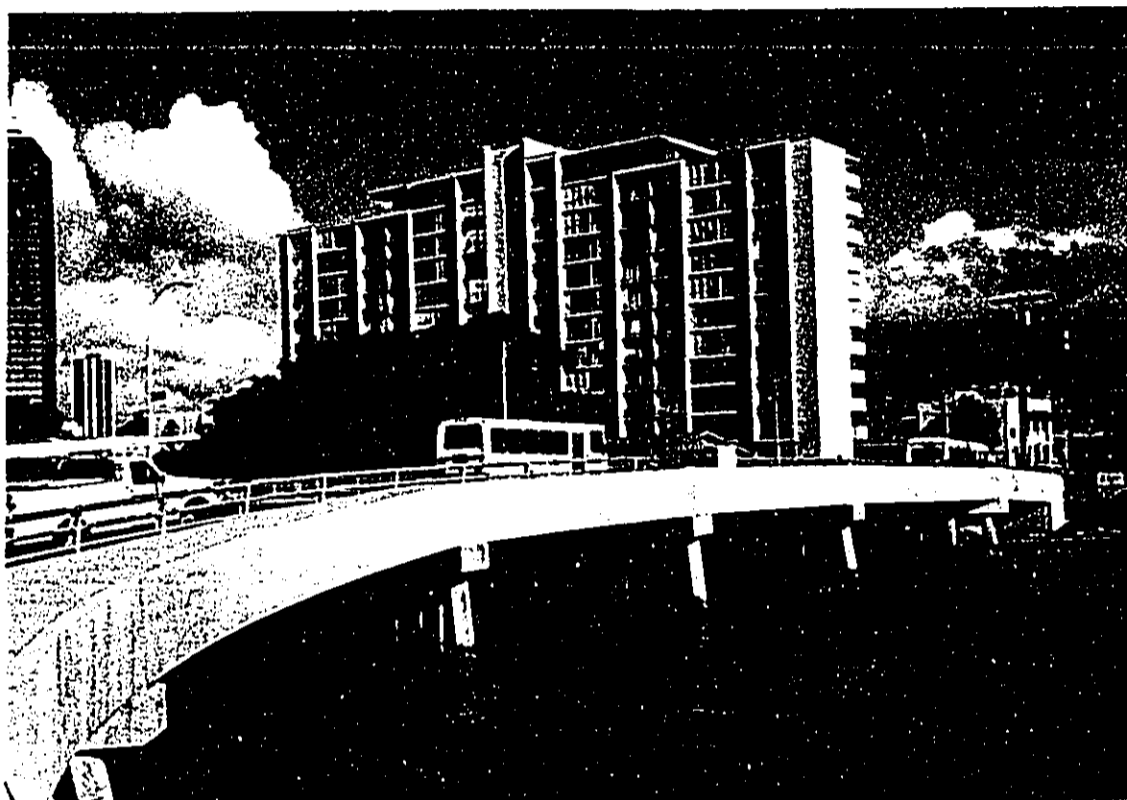
Figure 11: (bottom) Date Street Bridge, looking SW.
