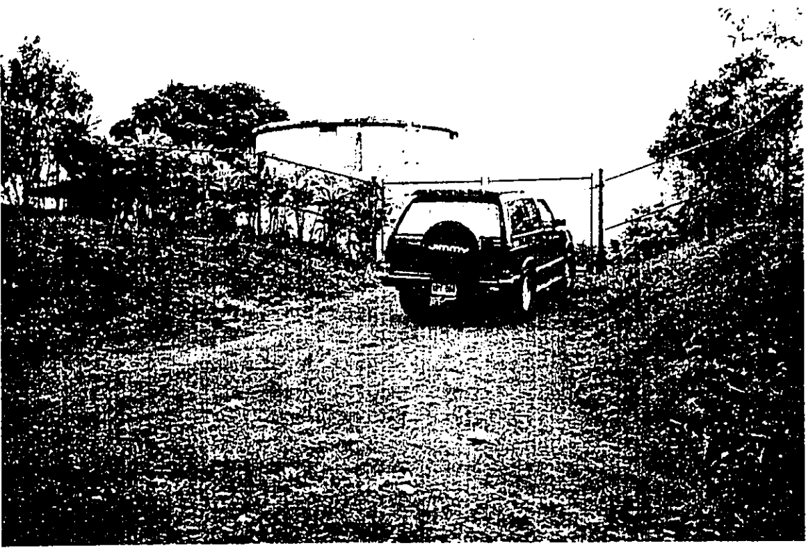
View west at entry to Makapala reservoir site
