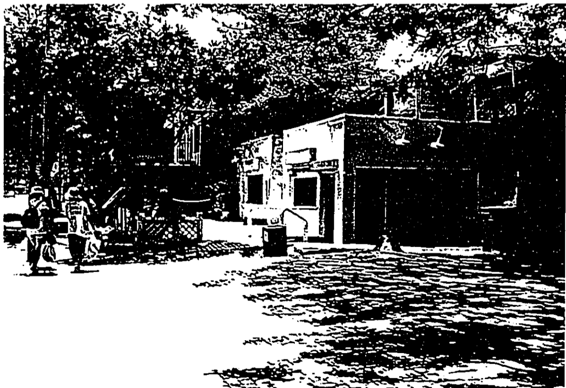
Figure 11 Concrete buildings on Kuhio Ave.; view southeast
