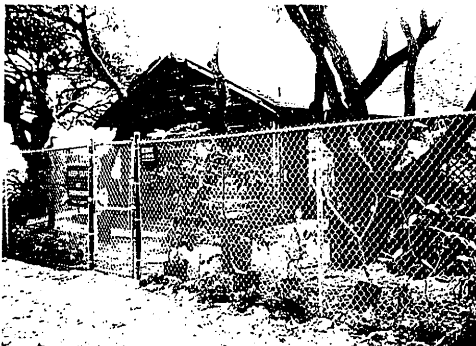
Figure 20: View of Caretaker's cottage and chainlink fence from the walkway Figure 21: View of walkway, chainlink fence, and construction tape barrier.
