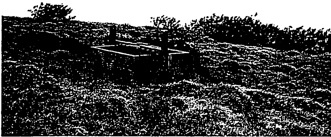
Photo 8. Concrete trough located above the Maui wind turbines project area, view to southeast.
