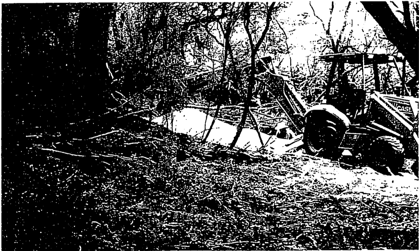
Photo 12 - Excavation in process, BT 4. Site 4467 in background.
