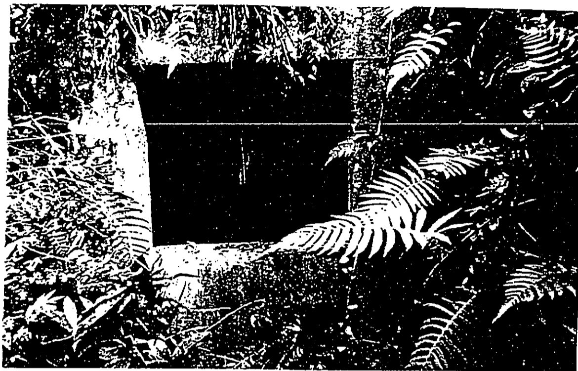
Figure 13 View of Entrance to Portal # 4, View to North West
