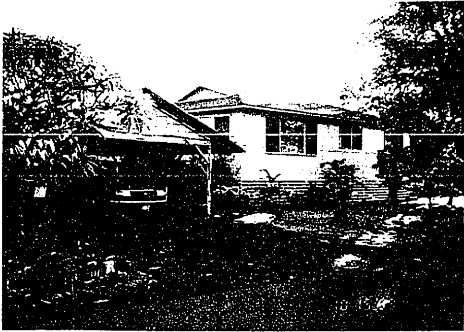
6. The existing single family dwelling on Parcel 8 serves as a QLCC caretaker's cottage and will remain in that use. The house and garage/storage room consist of 1,840 sq ft.
