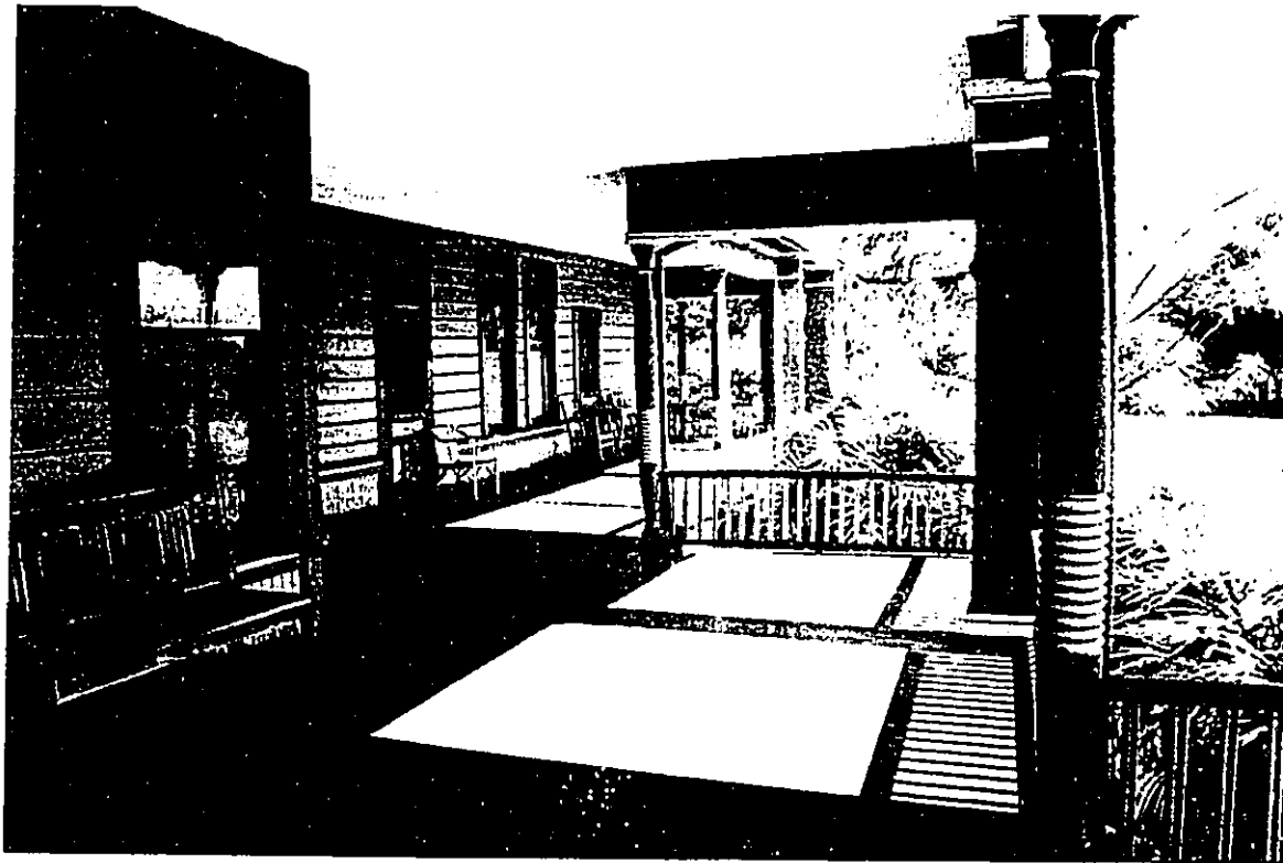
Photo 19 (top) - Front lanai Photo 20 (bottom) - Damaged flooring at lanai
