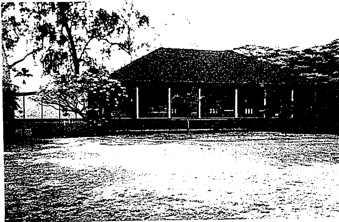
Figure 71 Site 50-30-9-764/B: Photo of guest house. View to northwest.
