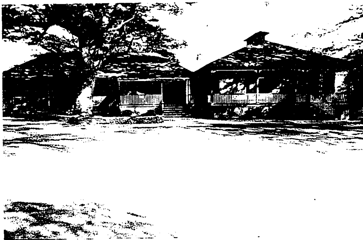
Figure 72 Site 50-30-9-764/C: Photo of servants quarters. View to southeast.
