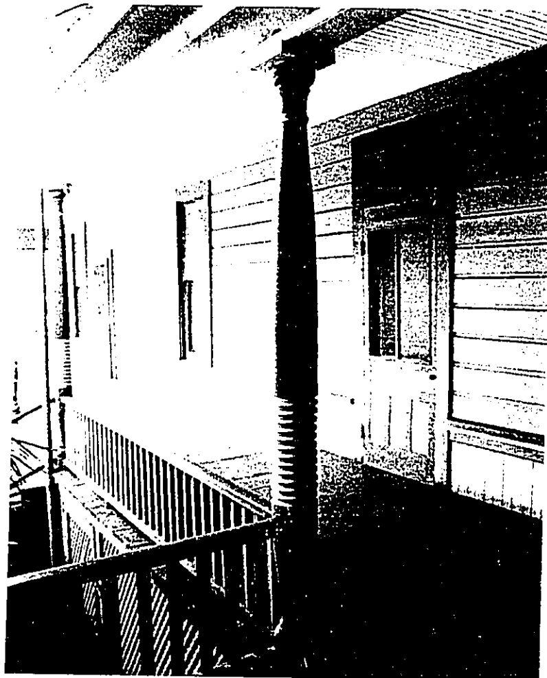
Photo 21 (top) - Decorative wood column at courtyard Photo 22 (bottom) - Deteriorated column top at courtyard
