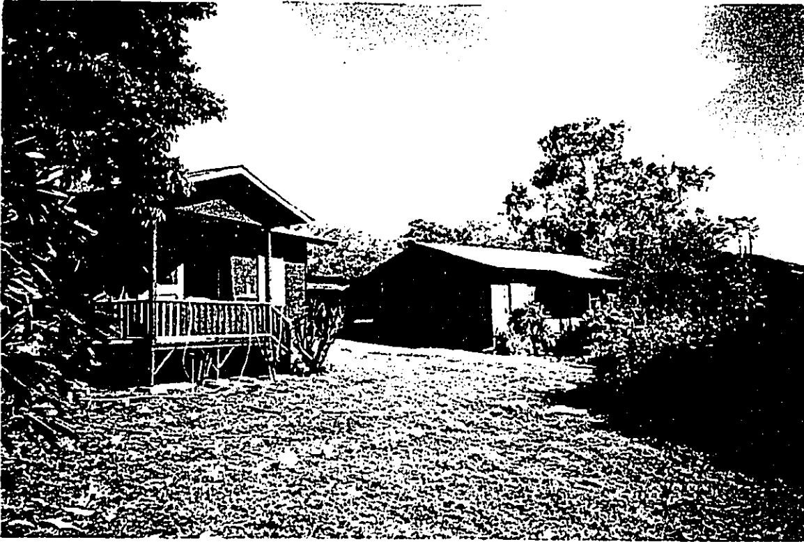
Figure 53 Workers camp houses.
