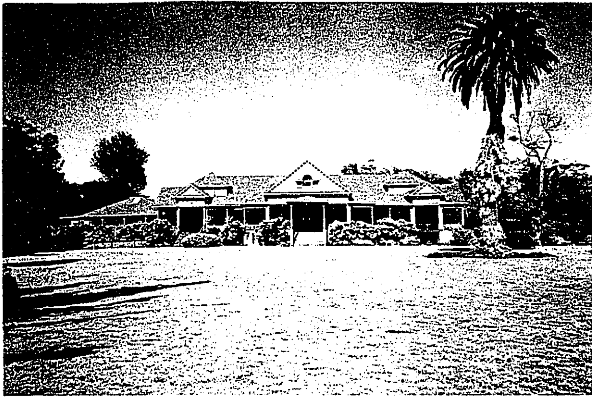
Figure 67 Site 50-30-9-764/A: Photo of front of main house. View to northeast.
