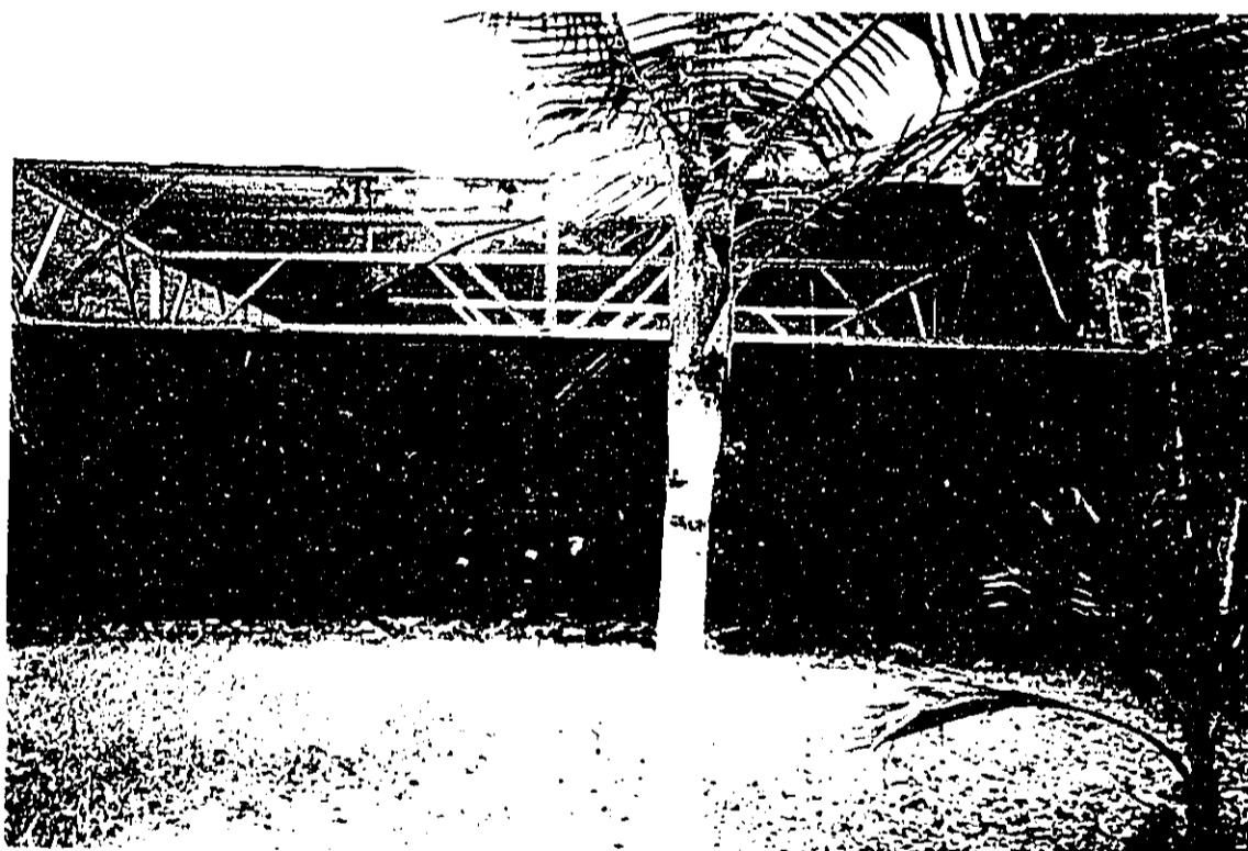
EXHIBIT E-2 TEMPORARY SHADE CLOTH STRUCTURE PARCEL (3) 8-3-05:7
