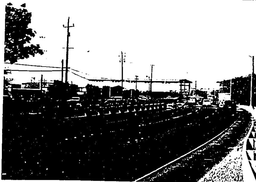
Photograph 6. Ewa View of Maintenance Facility From Nimitz Highway Near Ala Kawa Street.
