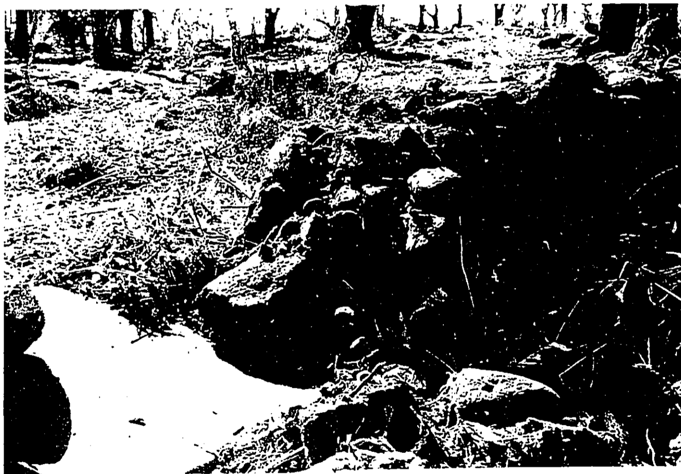
Photo 3 - View to the southeast of collapsed portion of Feature A wall. Note concrete walk in lower left corner of photograph.
