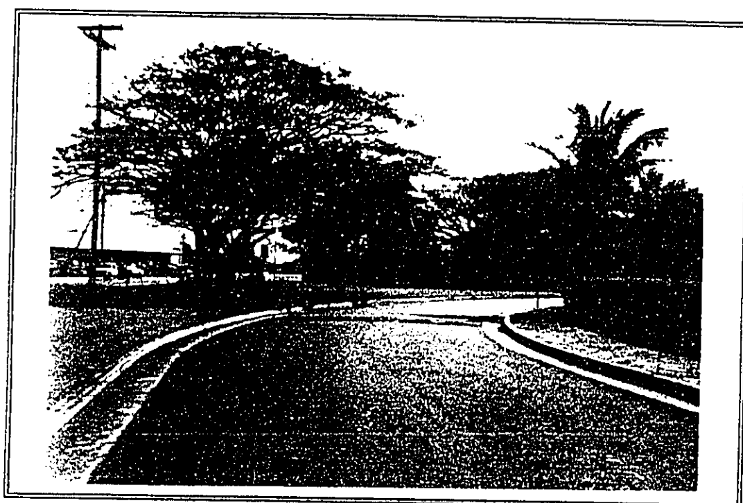
Photo 6: View looking to the east in the area of the proposed clarifier modification area. Sand Island Road Parkway is on the left.
