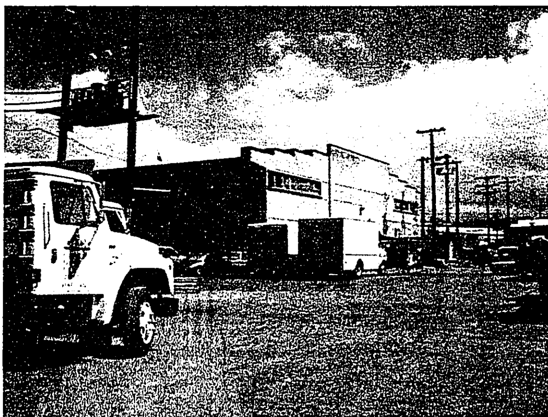
Building 905 Photo b
