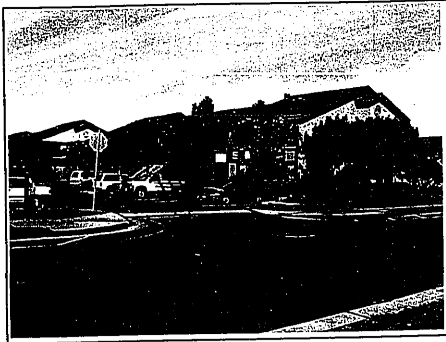
The Haleakala Gardens apartment complex is situated across Kulanihakoii road and is within 500 feet of the subject property.
