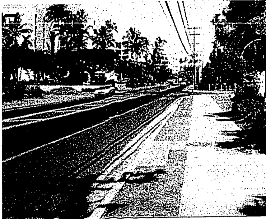
Figure A-1. Looking north along South Kihei Road toward Kulanihako'i Road
