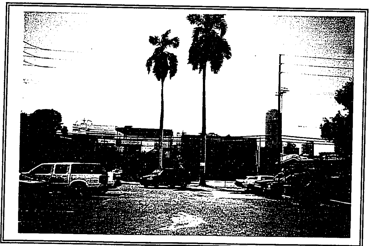
Photograph No. 2 View from 1828 Young Street Looking South Toward Young Street
