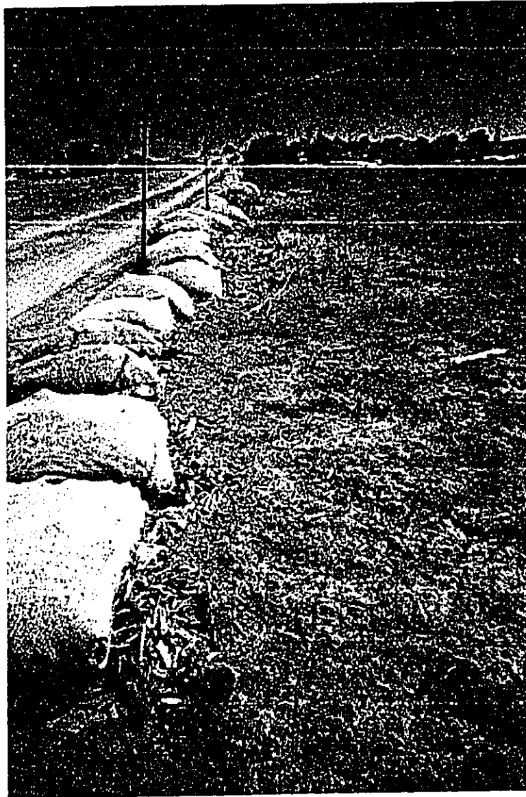
Figure 4-2 Existing Erosion Control Along K-1 Service Road
