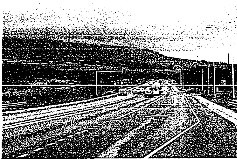
Intersection of Piilani Highway and Ke Alii Alanui Looking South
