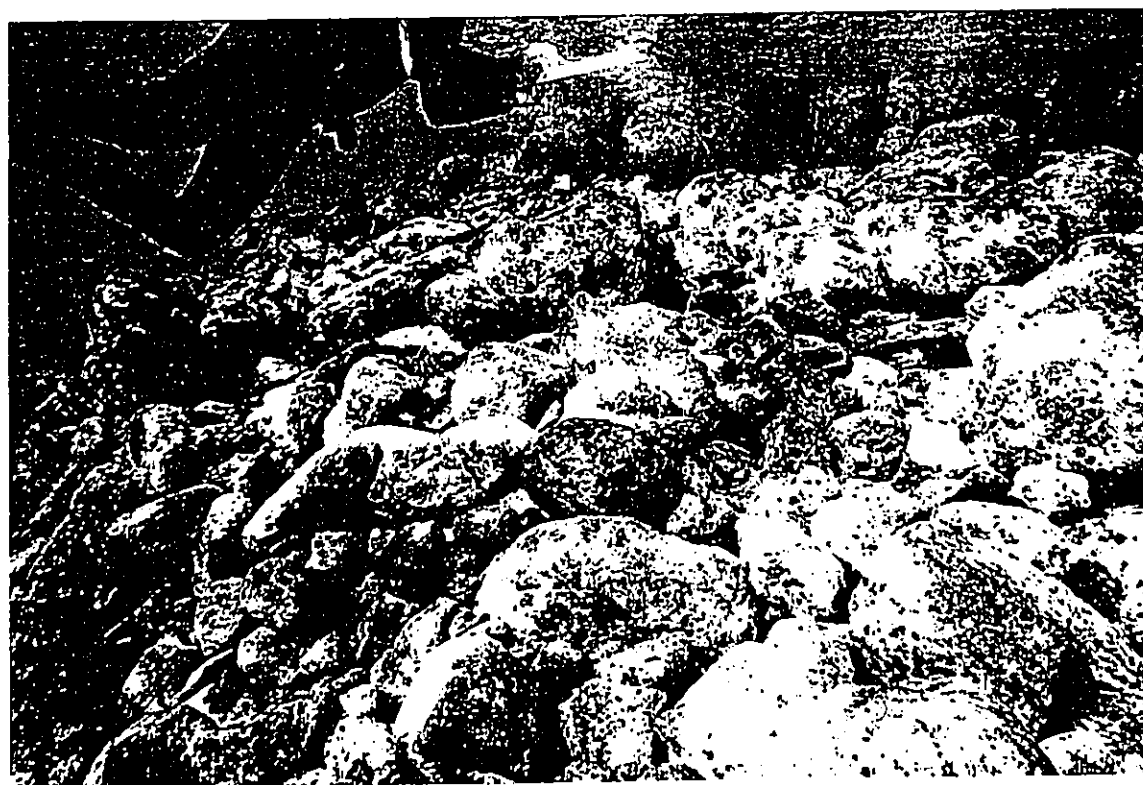
Figures 2 and 3. Two views of boulders located on inside edge of existing breakwater at Kaumalapau Harbor. Water depth is 1-2 meters. Photos courtesy of J. Naughton, NMFS.
