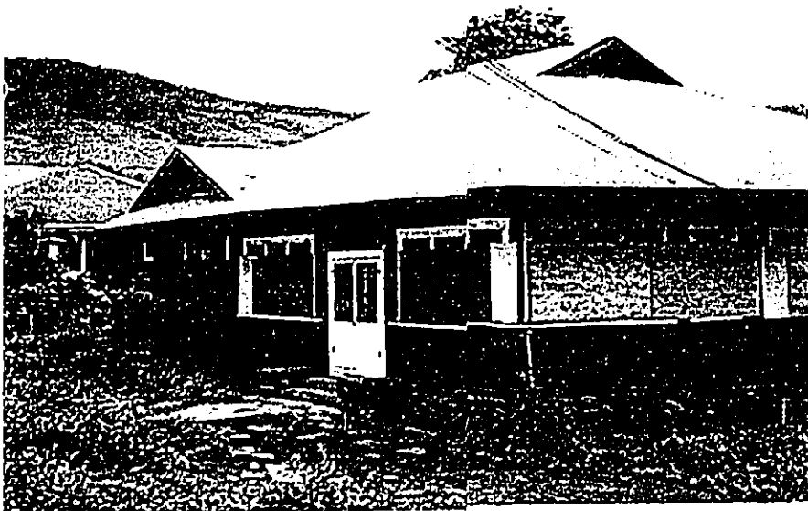
3. Abandoned Duplex (Building "C")
