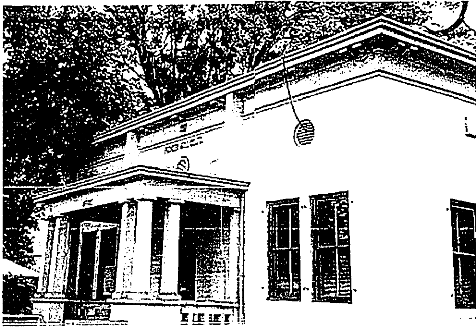
1. Pioneer Mill Administration Office Building (Building "A")
