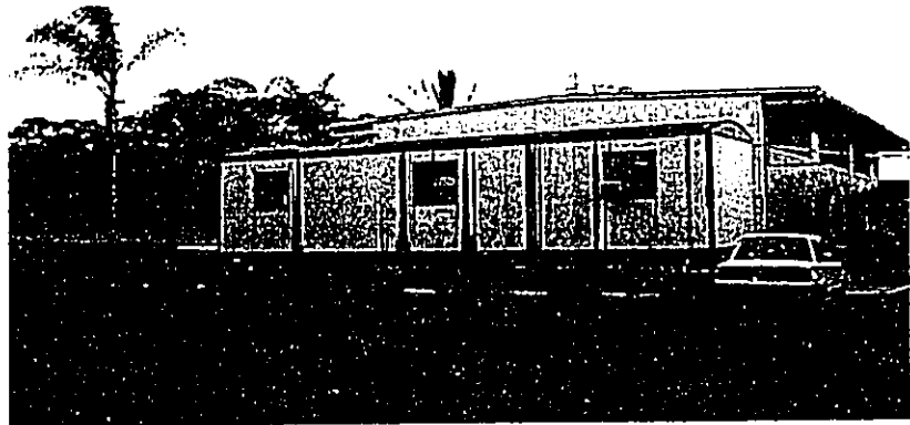
Photo 8 View Of Temporary Trailers Used For Facilities
