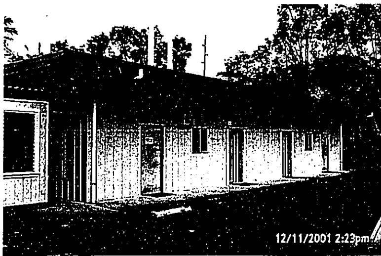
Photo 3 View Of Building At PBARC's Stainback Facility
