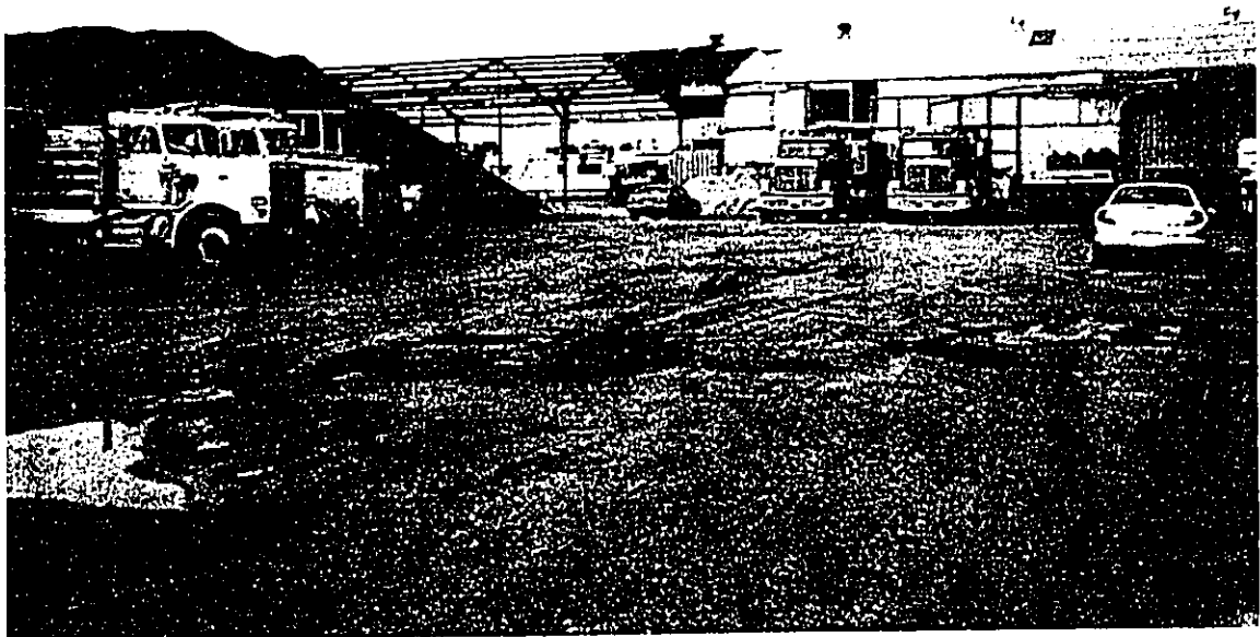
Figure 3 The site of Middle Street Transit Center expansion project is currently a truck depot with little or no wildlife habitat. Kalihi, Oahu, Hawaii. December 2001
