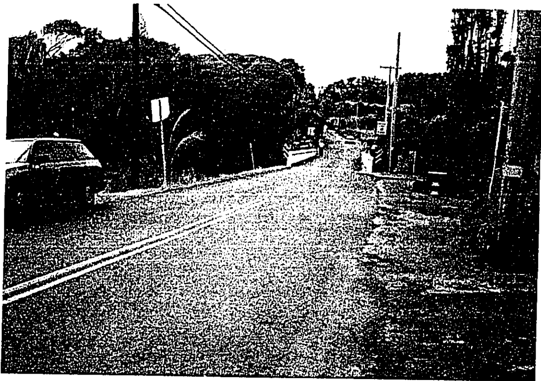
Photograph 2: View of Waiohonu Bridge looking south-west towards Kipahulu
