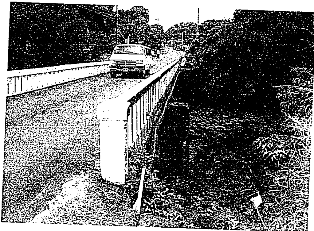
Photograph 12: View of the upstream side of Waiohonu Bridge looking south-west towards Kipahulu
