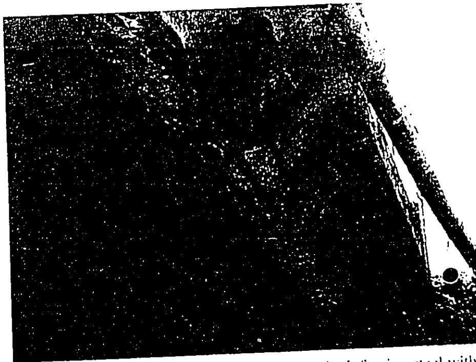
Abutment #1, honeycomb, water stains, rust stains, efflorescence, mold, mildew, scaling.
