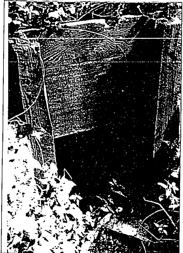
Figure 2. This wooden gate with an opening about 1-foot by 1-foot is used to control water from the main stem of the ditch to the end user - a grower of sweet corn. The second road crossing is over the concrete pipe culvert immediately behind this gate.
