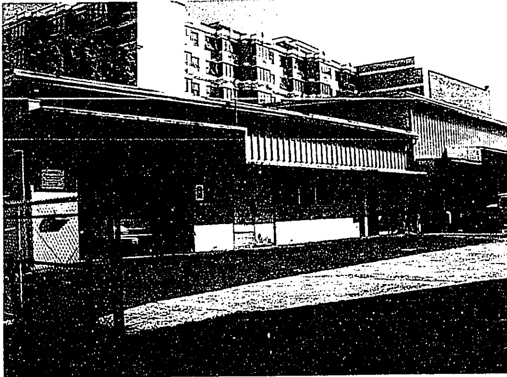
Image 3. Maintenance Building to be Demolished for Parking Lot.
