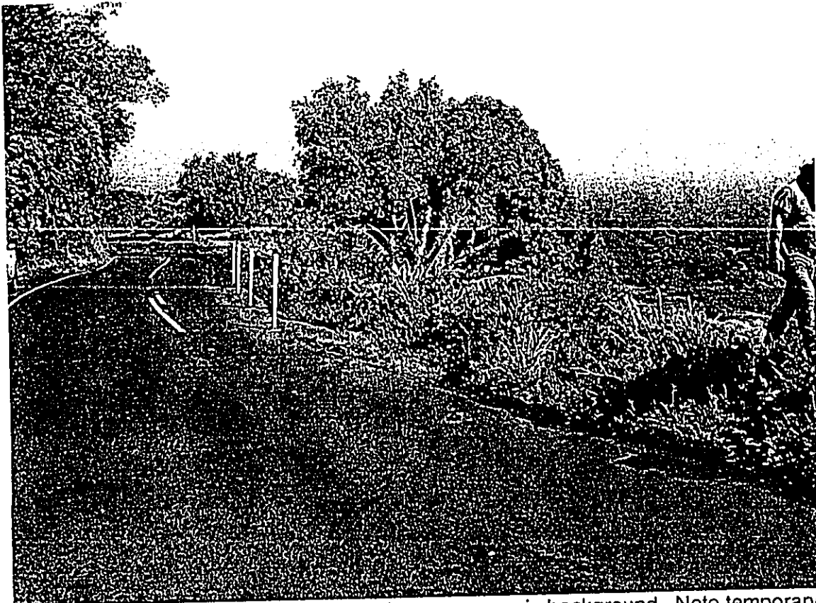
View of site, looking northeast towards Keanae, ocean in background. Note temporary pylons to direct traffic away from hazard area. Grouted rock wall two feet in height on highway side. Photo courtesy of DOT.
