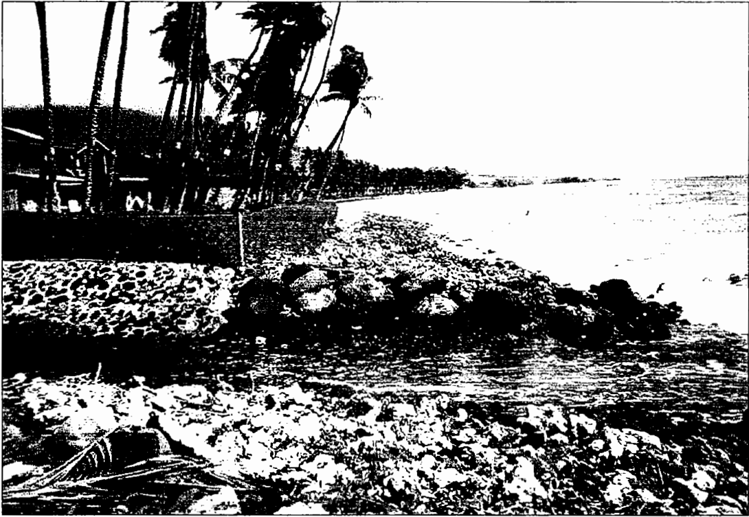
Figure 3-1 – Kau'aula Stream Outlet at Makila Point
