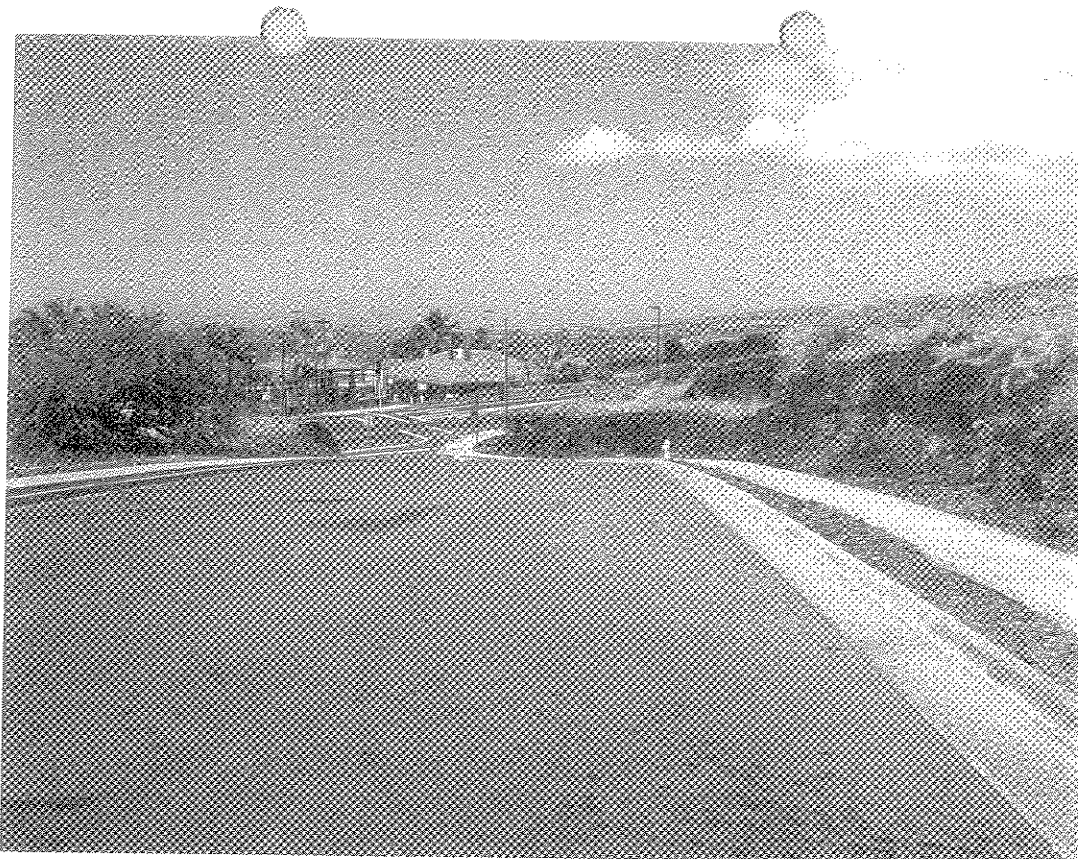
View of Project entry roadway connection built to County dedicable standards.
