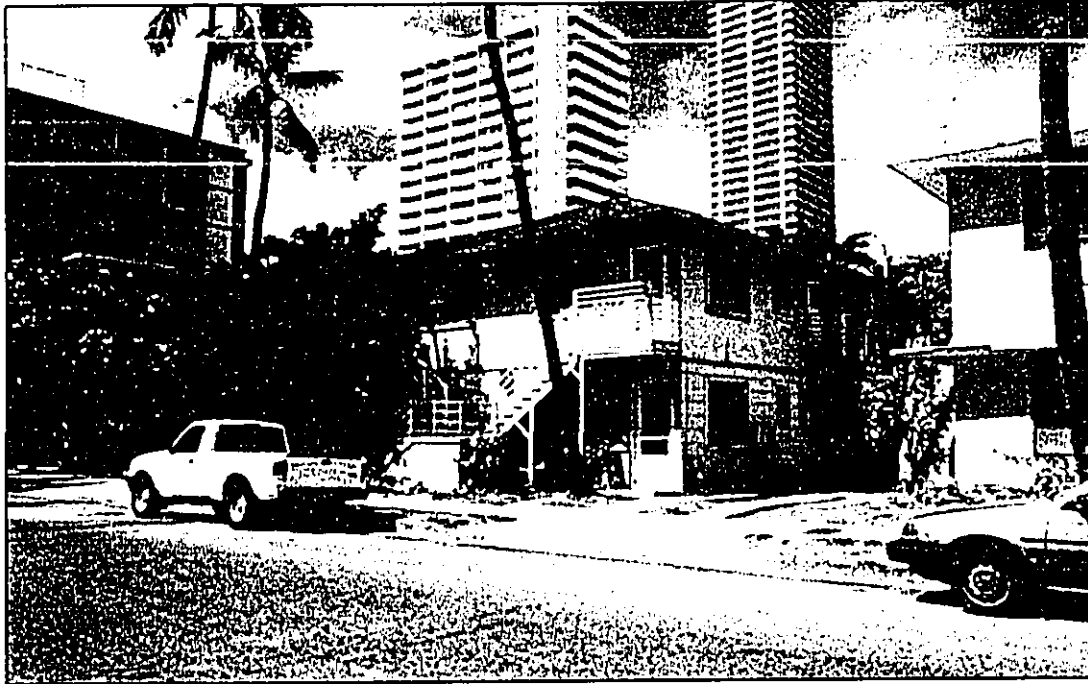
Photograph 15: 434 Launiu Street, two-story apartment building located across the street from the project site. (Reference item No. 13 in Figure 3).
