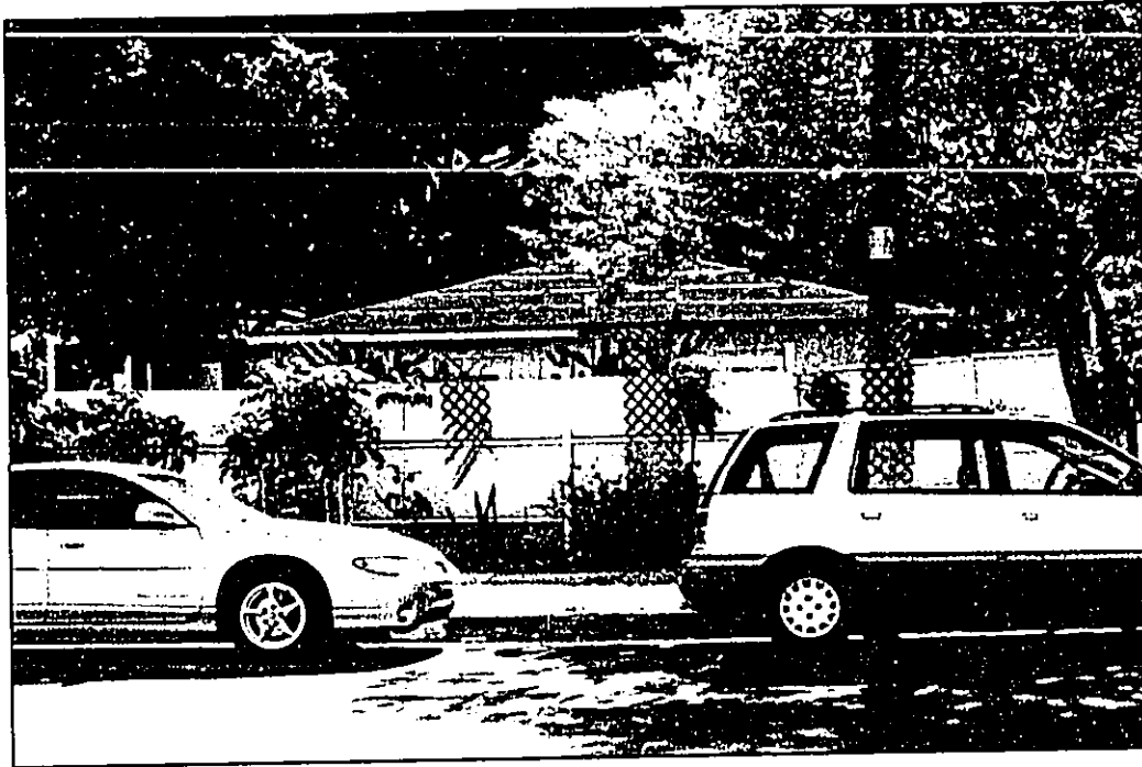
Photograph 3: Existing single-family home. (Reference item No. 3 in Figure 3).
