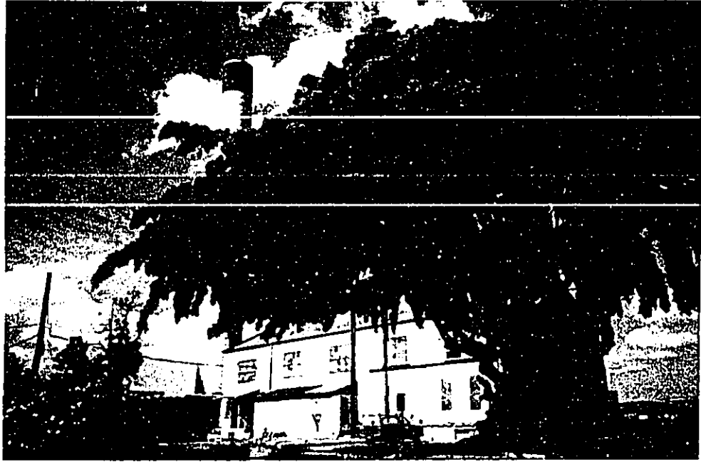
3) The former Oahu Sugar Company Generator building will be renovated and expanded to provide space for fitness activities. The old mill smokestack will be retained as a reference to Waipahu's history and cultural roots as a plantation town. The large banyan tree will be retained.
