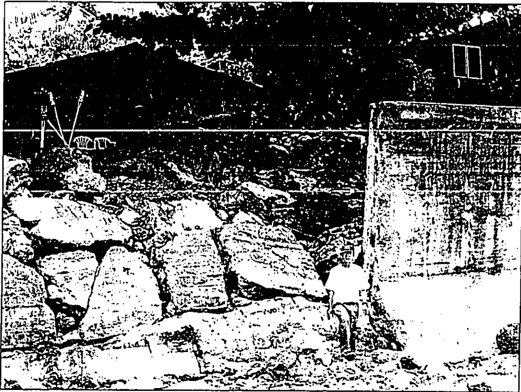
Figure 5. Collapsed wall at 59-601 Ke Iki Road.
