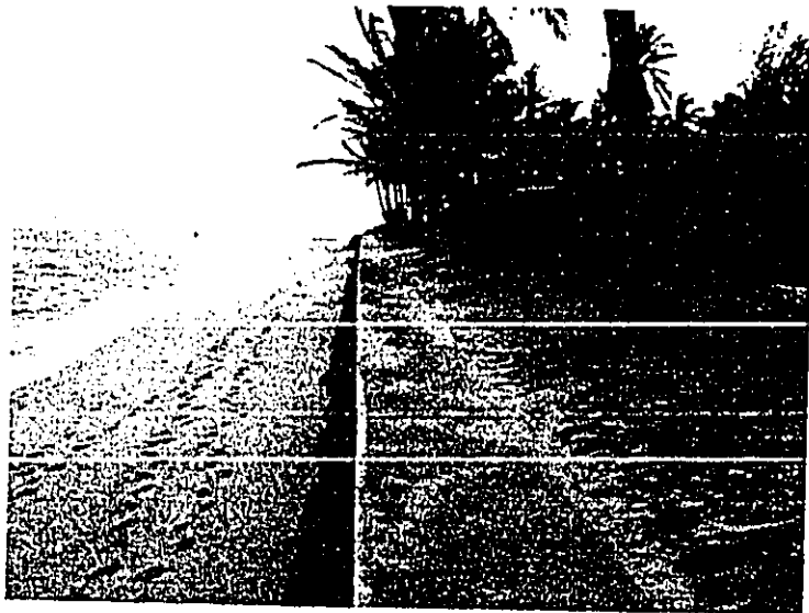
View eastward along the top of the seawall fronting the Mokuleia Beach Colony. Note the narrow beach.
